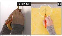
Measure and mark the location where panel will be placed and mark the orientation on the back of the panel.
