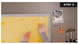
Insert reusable marking plugs into the Snap-On anchors.
